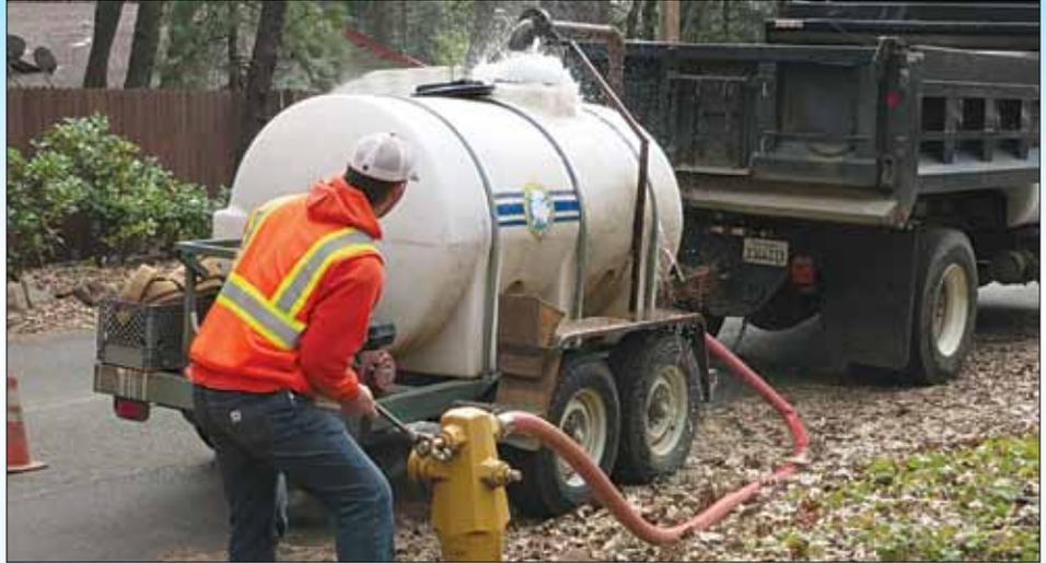
**GETTING THOSE PIPES FLUSHED OUT**—A Paradise Irrigation District employee finishes flushing out a hydrant in central Paradise in February. If the "flushed" water would damage landscaping or overwhelm the roadway, the water is flushed into a water tank and then released in a better area.
